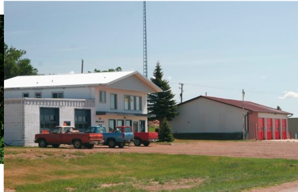
RM #12 Office and Fire Hall
